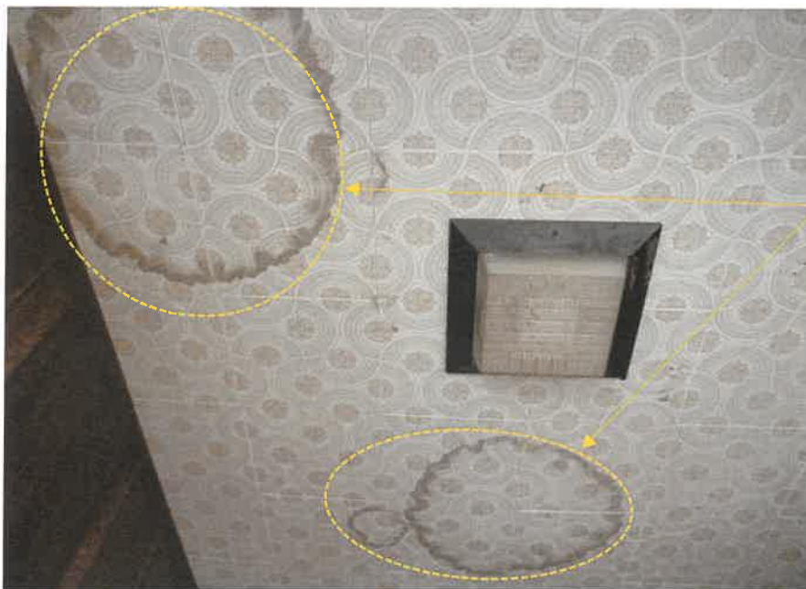
⑤玄関天井
