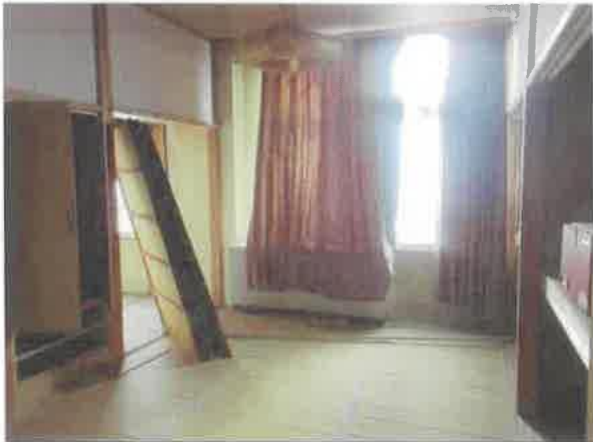
No. 18 物件8・9:3階 南側和室の状況
