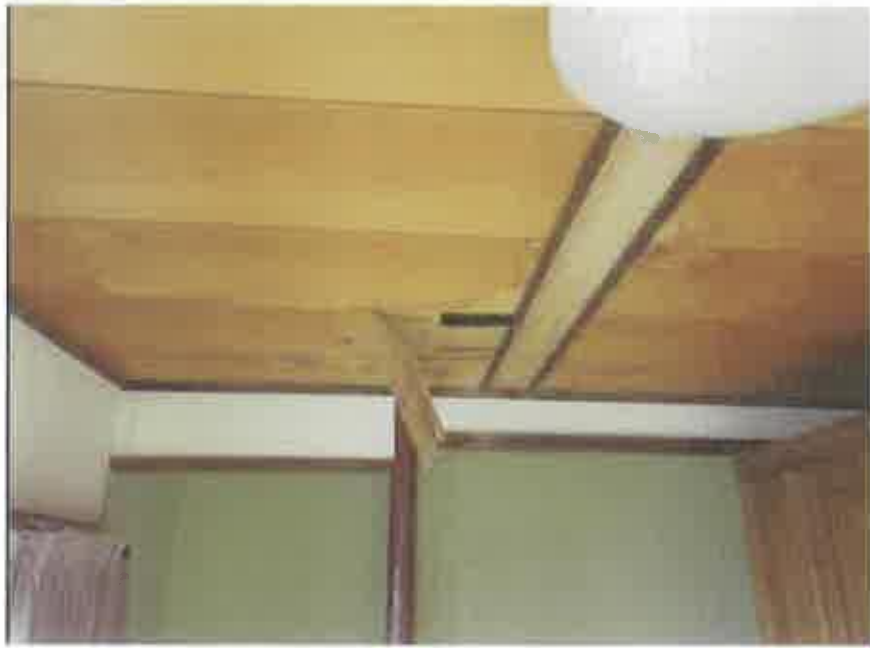
No. 17 物件8・9:3階 和室(301号室)の天井の状況
