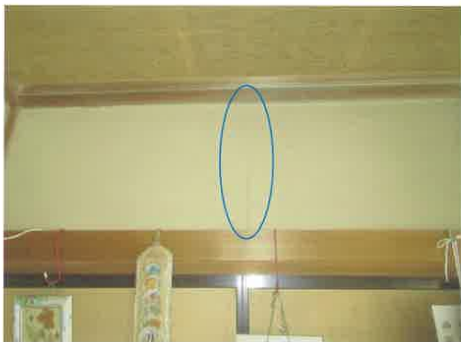
物件2:和室2内壁の亀裂
