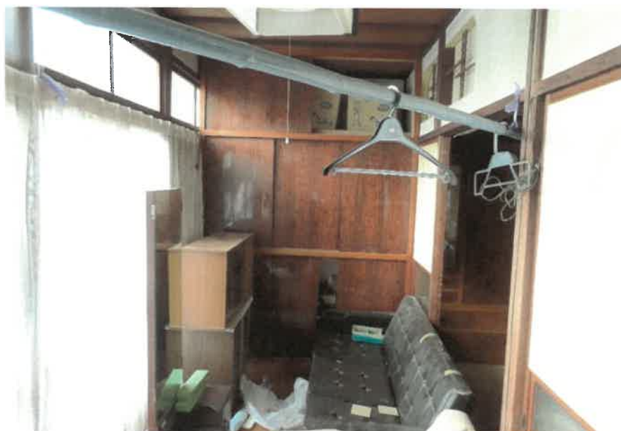
物件2:1階広縁の状況
