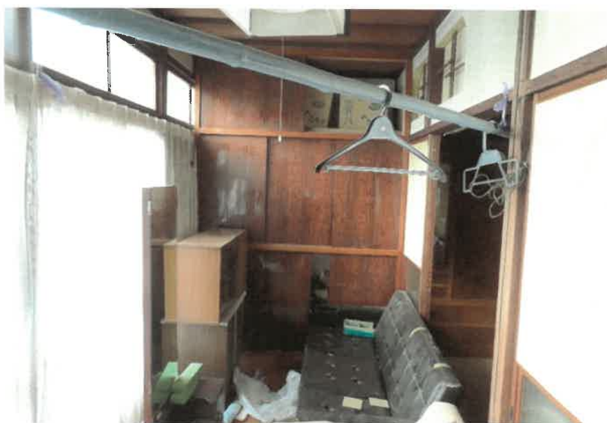
物件2:1階広縁の状況
