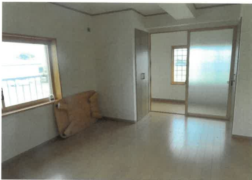
物件3:2階洋室(南東角)の状況
