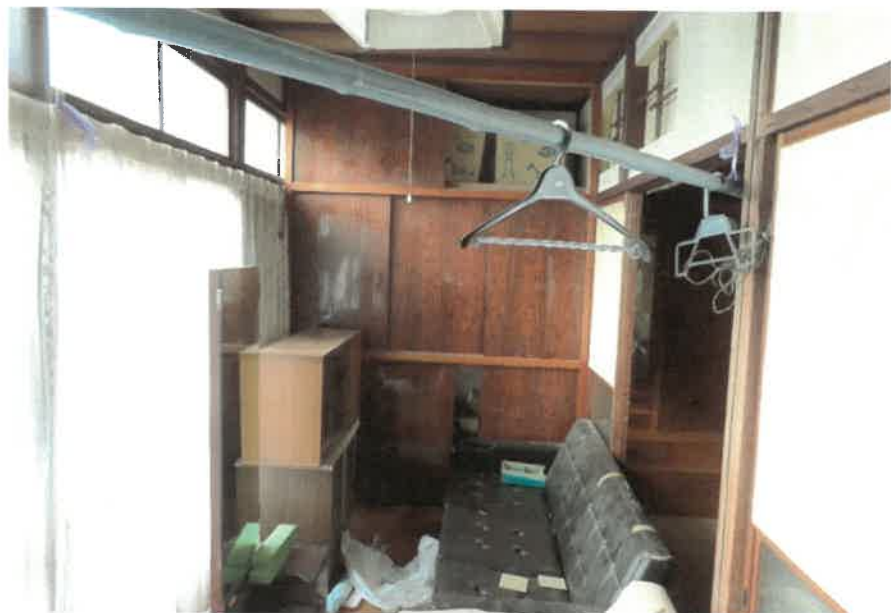
物件2:1階広縁の状況
